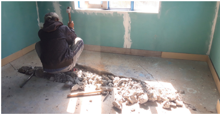
Jamyang working on leveling the floor in Alexi's bedroom, Shanti Bhawan, Kullu-Manali valley, India
